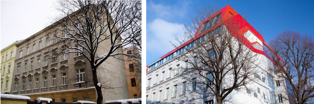
Object Wißgrill Alley before and after comprehensive reconstruction and attic expansion (Photos: Ulreich, Gassner & Partner)
