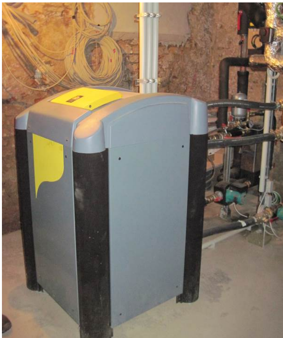
Eberl Alley: Groundwater thermal pump and extraction well
